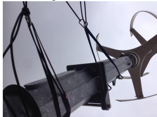
Photo 60 Slings around a wind turbine
