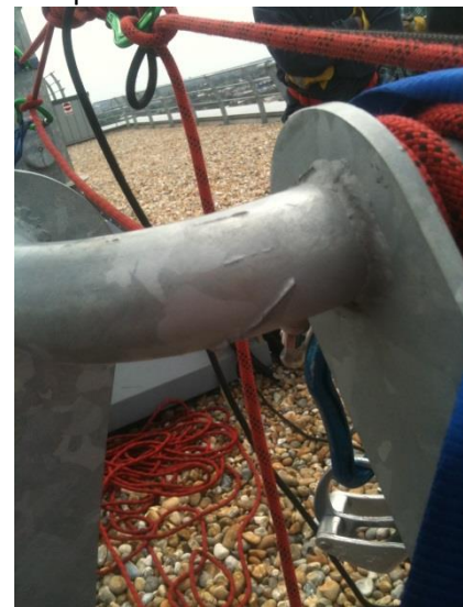
Photo 32 A burr on the underside of a perimeter fence
